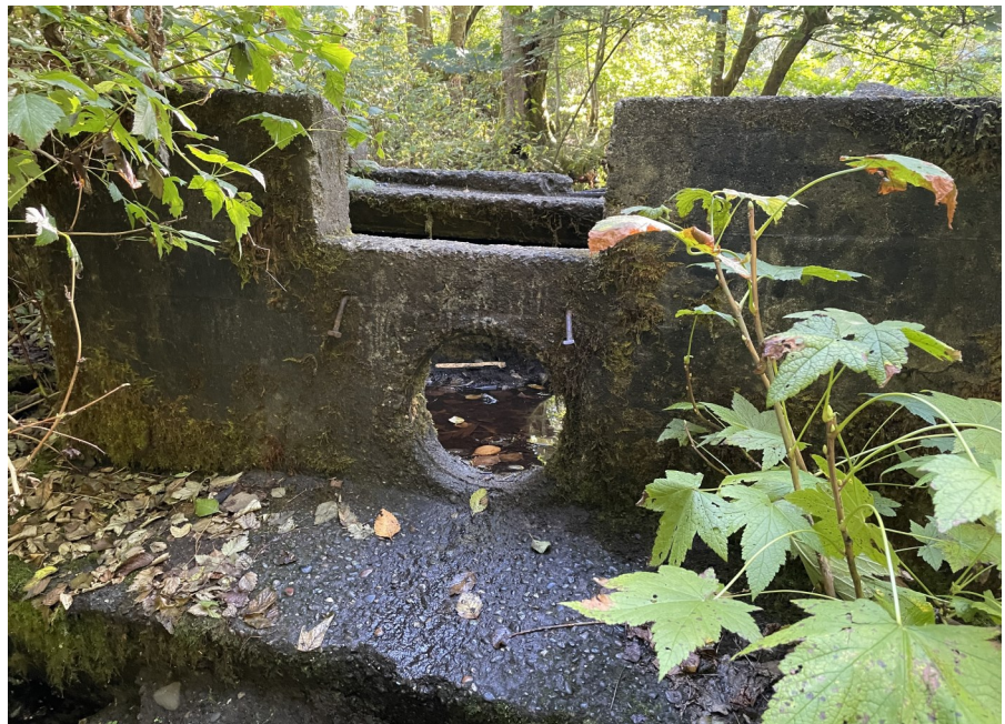
The weir directed the Shell Creek flow into a pipe which fed into the main water system comprising an underground water main running west on Main Street. Homes and businesses could tap into this main for domestic water supply. (photo Sam Spencer)
